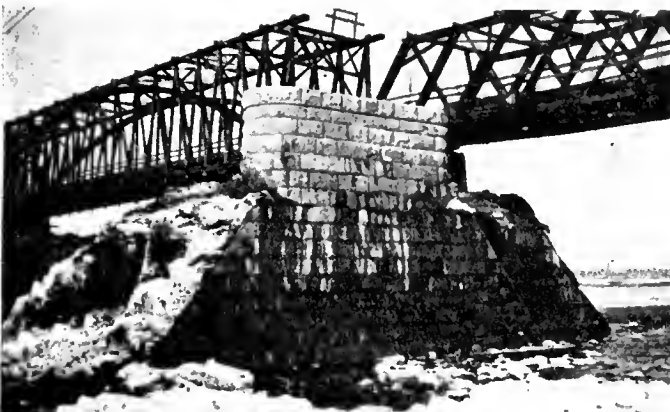
Fig. 3.—Pier No. 4 completed.
